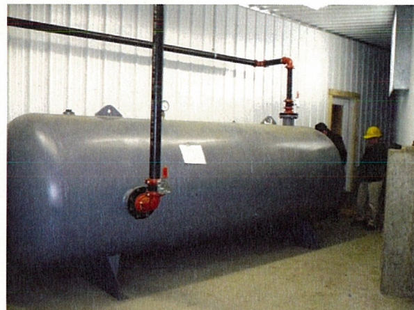
2,120 gallon air receiver (compressed air storage tank)
