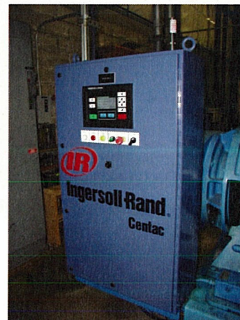
New air compressor control cabinet
