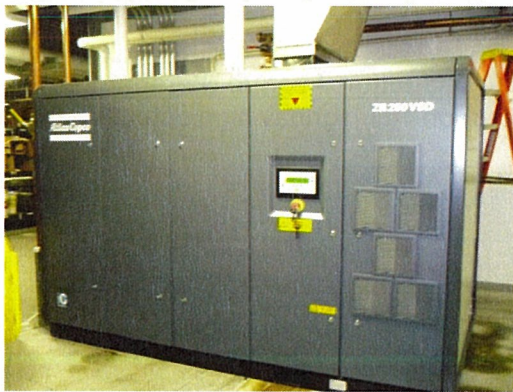
350 hp water cooled air compressor
