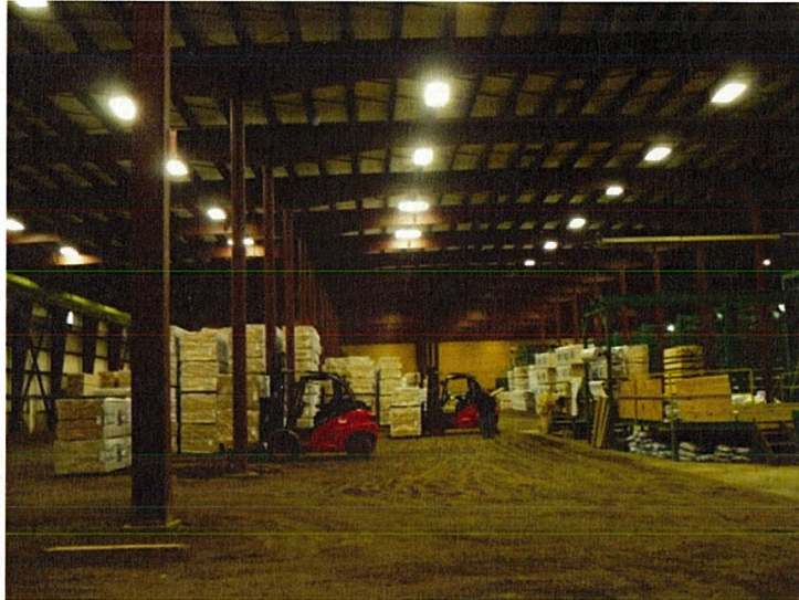
Lumber storage area with new highbay high performance T8 lighting fixtures
