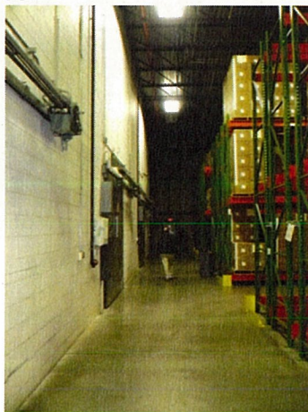
High Output T5 Fixtures with occupancy sensors
